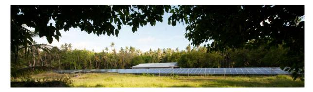
This large solar photovoltaic/diesel hybrid mini-grid system, installed on Fakaofa, one of the three atolls that make up Tokelau, delivers over 90% of the atoll's electricity needs from renewable sources.
