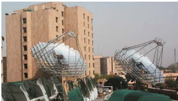
Solar Thermal System for Steam Generation at ITC Hotel, New Delhi
