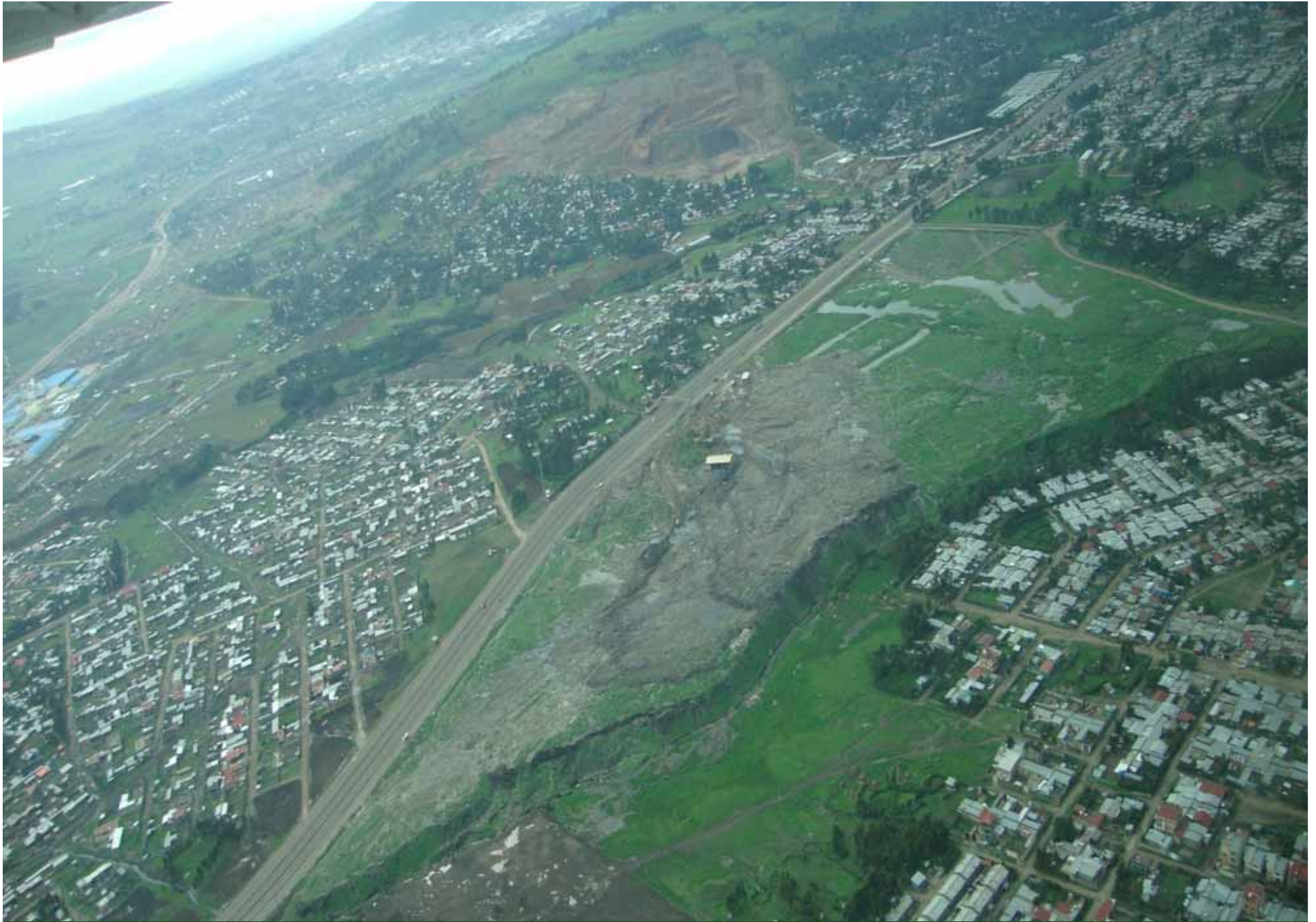
Aerial View of Reppi /Koshe Solid Waste Disposal Site, Addis Ababa, Ethiopia
