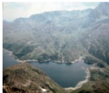
Fig. 2. Lake Lanoux, in French Sardinia, whose utilization is regulated by a Franco-Spanish Commission and which provided water supply for the white water rafting competitions in the 1992 Olympics Games held in Barcelona.
