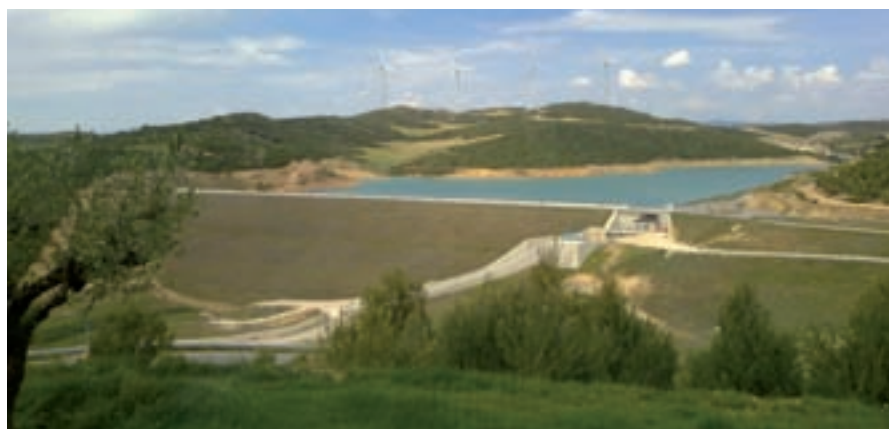
Fig. 6. Irrigation facilities. Navarra canal.
