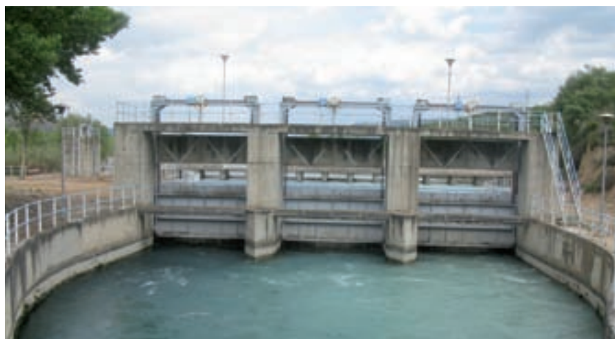
Fig. 4. Hydroelectric users' infrastructure. Arias canal (River Cinca).
