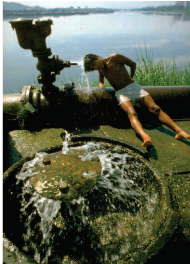
Fig. 5. Nicaragua water pipes. Source: WHO.
