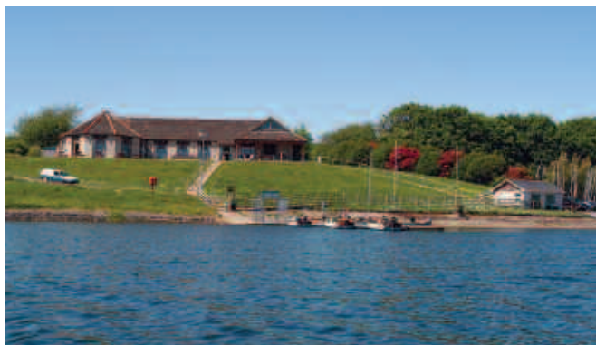
Fig. 6. Bristol Water. Dam Chew valley. Bristol, London.
