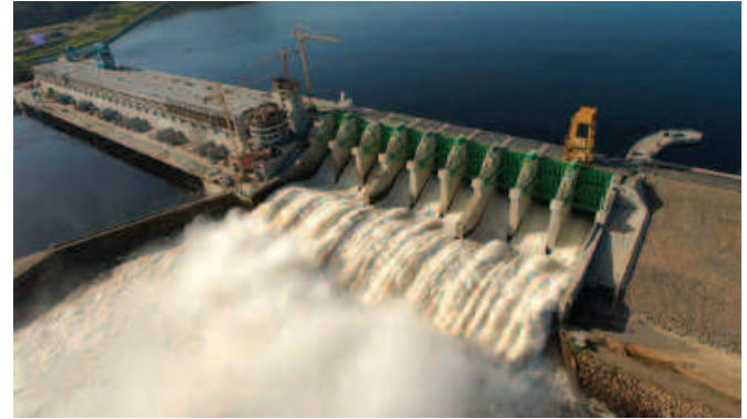
Fig. 11. View of the Caruachi dam and hydroelectric power facility (Venezuela). Energy production. 2,160 MW. Source: Dragados.
