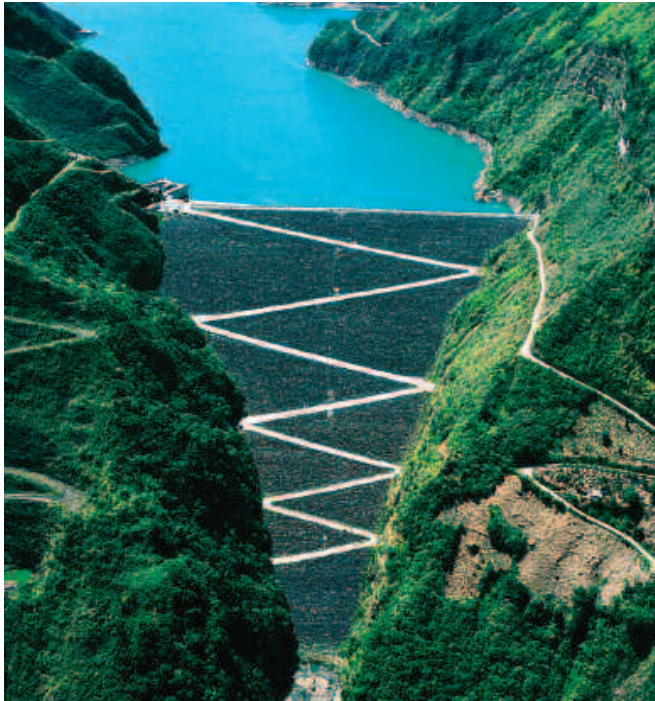
Fig. 10. Guavio dam (Colombia). Energy production. Rockfill dam with impervious core; height, 247 m, reservoir 1,140 hm 3 . Plant, 1,600 MW. Source: Acciona and Endesa.
