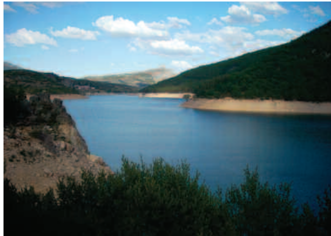
Fig. 5. Storing water when there is surplus in order to supply it when needed is the key to meeting demand and creating a favourable environment for development. The Compuerto dam and reservoir, Carrión river, Spain.
