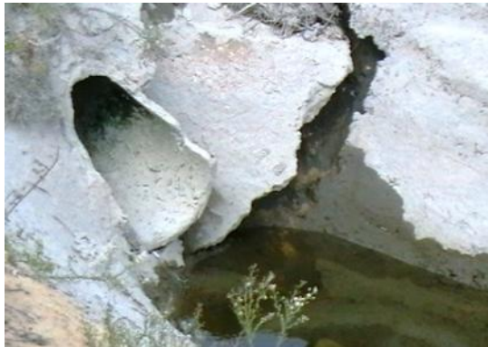
Inlet of mesqa over the outlet of canal (Photo 7) -
