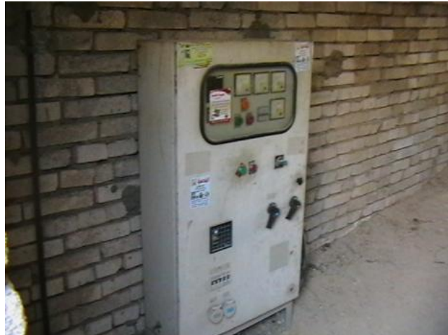
Transformers (Photo 10) – Control panel of Irrigation Motor (Photo 11)
