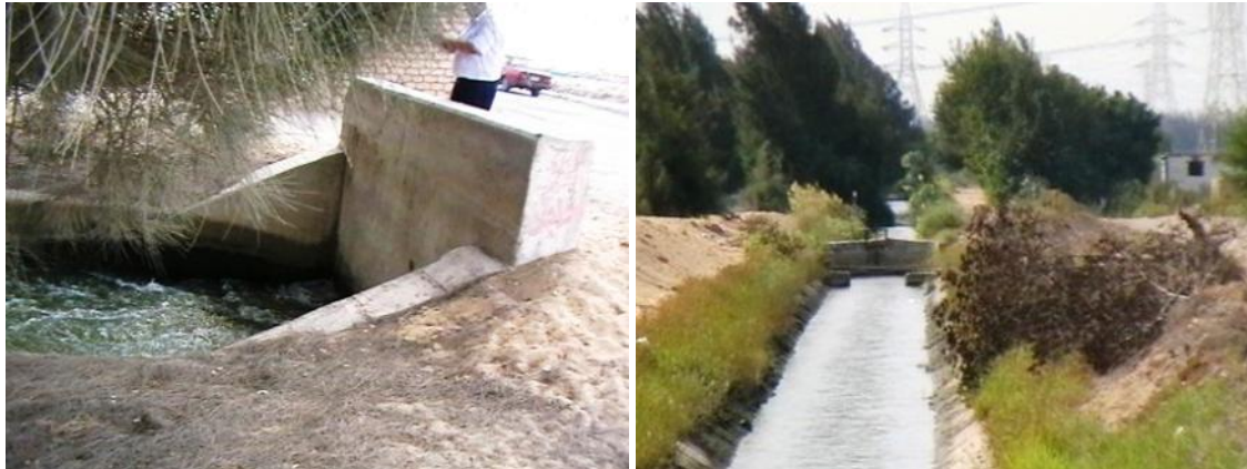
Reverse slope of mesqa stream (Photo 5) - Constructions like barriers (Photo6)
